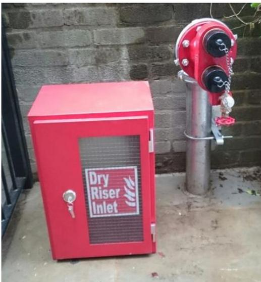
A dry riser is a system of pipe work and valves that runs up through a building. The system allows fire fighters to easily access water at a high pressure from each floor of the building. In normal circumstances these systems sit unused and can become damaged, neglected or even vandalised.
